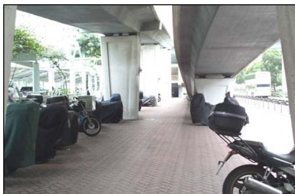
Possible Utilisation of Space under Footbridge
